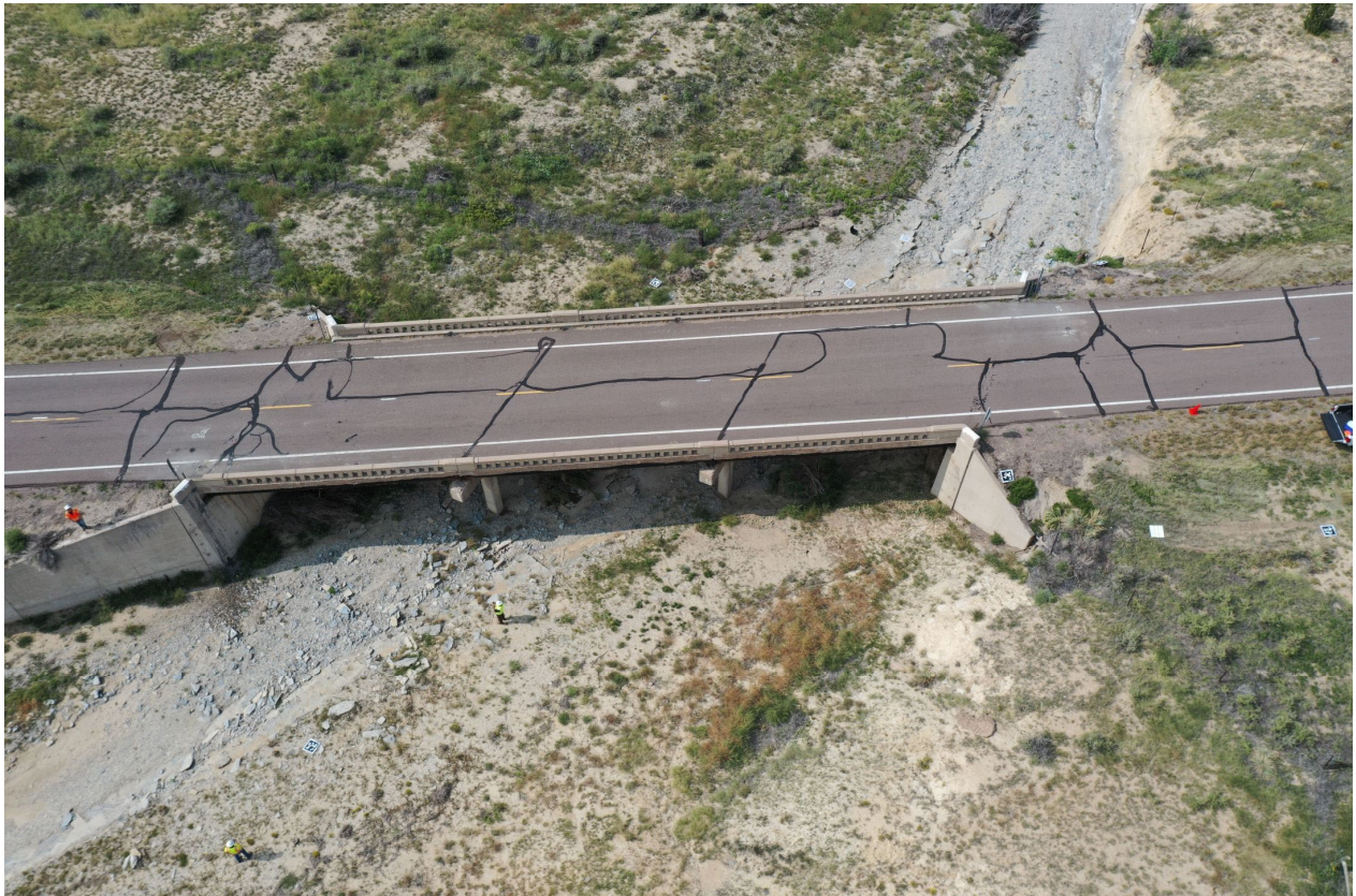
Picture 1 - Bridge M-21-C
