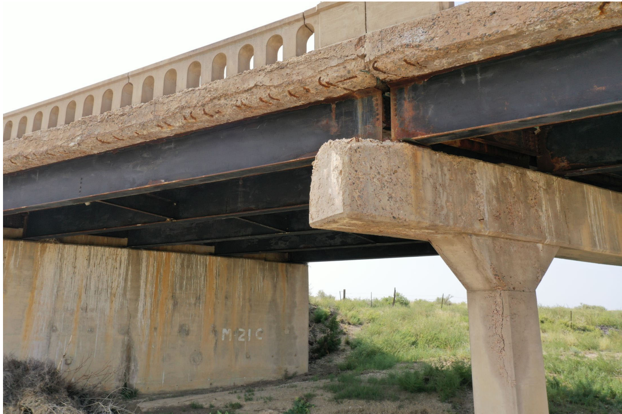
Picture 2 - Pier, Overhang, Deck, Girders
